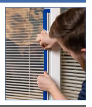
NOTE: If this is a single operator, run the tape all the way down the track.
