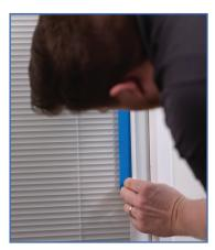
B) Continue this process until you reach the bottom of the track, working in small sections, ensuring that you have the track straight.
