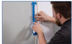
B) Continue down the vertical surface of the track toward the bottom. Once tape is applied, smooth the tape on the glass by running your thumb up, down and across the tape.
