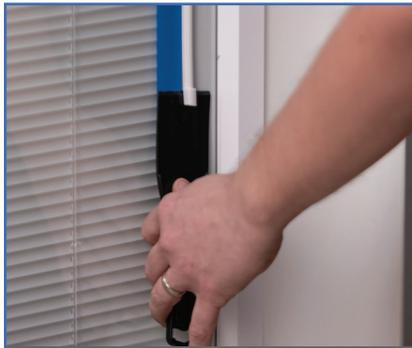
**B)** When you reach the operator, additional force will be required to free the magnets in the operator. To assist with this, pivot the track and operator 90 degrees and then pull away.
